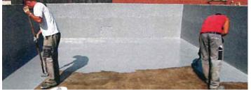
Using the high-pile roller (approx. 18 mm), roll the epoxy top coat AC 130R onto the dry primer AC 110 (consumption: min. 300 g/m<sup>2</sup> depending on the substrate, working time: approx. 20 minutes). The top coat AC 130R is designed for a high slip, chemical and mechanical resistance. Wait approx. 48 hours until using the surface (depending on temperature and humidity).
