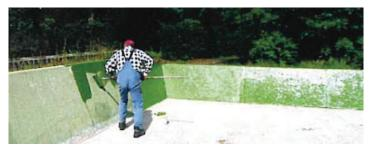
Using the high-pile roller (approx. 18 mm), roll the epoxy 2 in 1 top coat AC 122 onto the dry silo wall (consumption: min. 400 g/m<sup>2</sup> depending on the substrate, working time: approx. 20 minutes). The top coat AC 122 is designed for a high slip, chemical and mechanical resistance. Wait approx. 48 hours until using the surface (depending on temperature and humidity).
