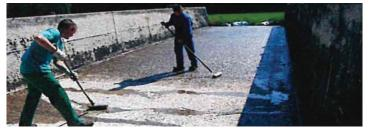
Using a high-pile roller (approx. 18 mm), roll the AC 110 epoxy primer onto the dry surface of the slatted floors and silo walls (consumption: min. 300 g/m<sup>2</sup> depending on the substrate, working time: approx. 20 minutes). The AC 110 primer does not only settle on the surface, but penetrates and anchors itself. As a rule, after approx. 24 hours, you can continue with the top coat AC 130R (depending on temperature and humidity).
